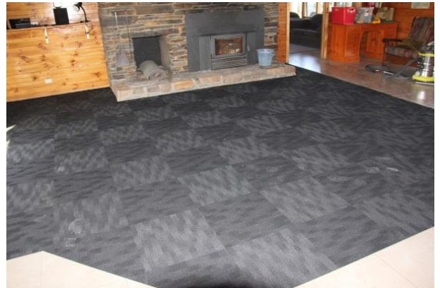
Carpet – the lounge area has been re-carpeted with durable carpet tiles, which enable the worn areas to be replaced easily – looks great
